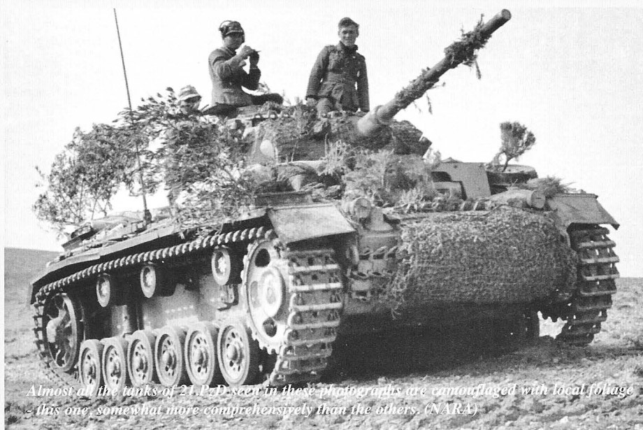
A Pzkw IV Ausf G (the Ausf F2 denomination was only used for a short time in 1942, Ausf G was the correct designation after that time. The suspension and power train were reaching their limits and designers could not up armour the turret front to the same level as the front hull (80mm), so it remained 50 mm thick to the end of production in 1945. (NARA)
