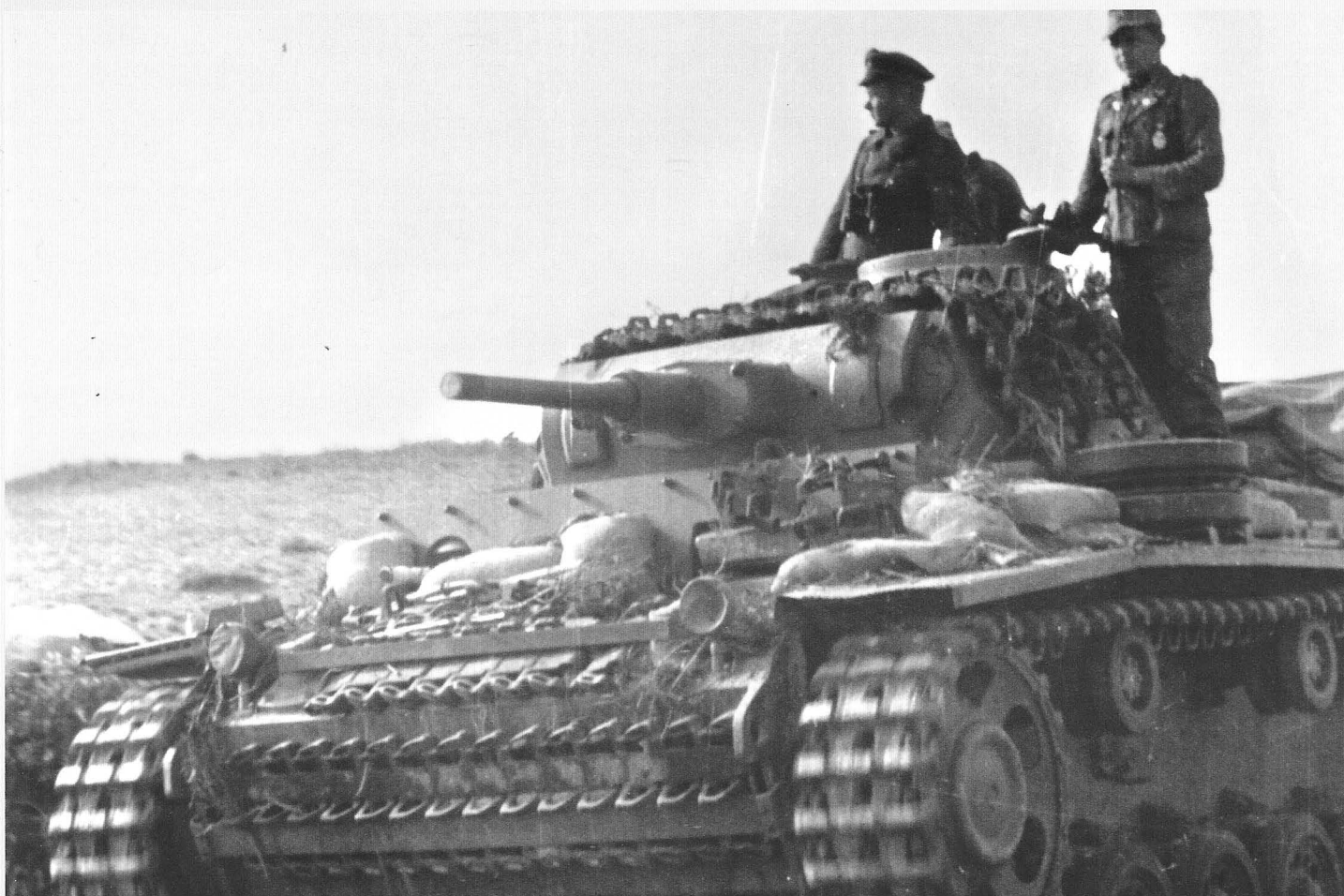
A rare variant of a Pzkw III Ausf J. A 20mm face hardened plate has been added to the hull front which was in itself uncommon on these short barreled variants. When this type of up-armouring is seen however it is usually applied to the turret front as well. It is possible that this tank had the plate retrofitted during an overhaul. Again, spare tracks and sandbags are used as additional protection. (NARA)
