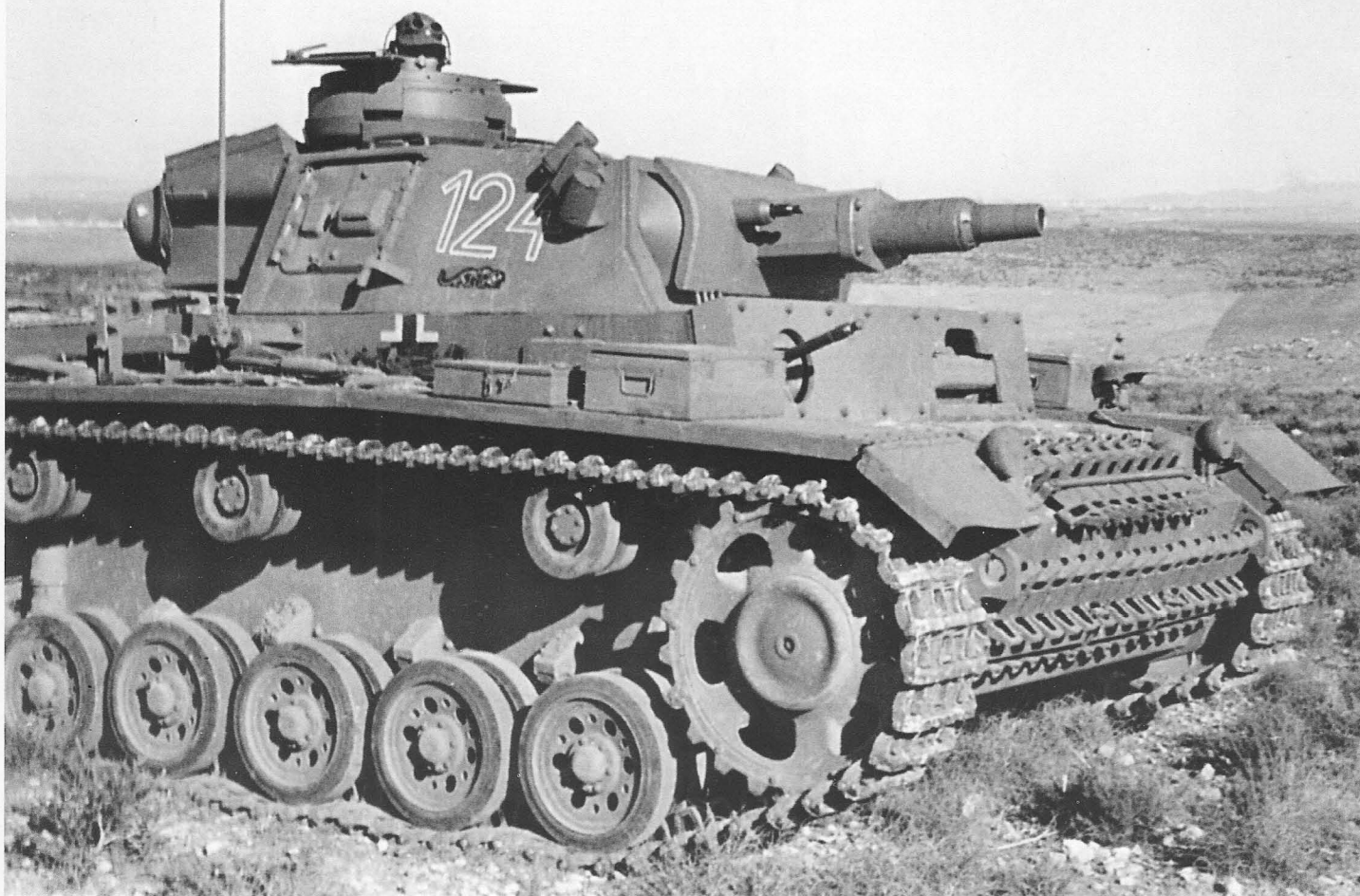
This Pzkw III Ausf N, No 124, is still brand new and in perfect shape. The desert bound-panzers were ordered to be painted in a two colour camouflage scheme of RAL 8020 with a disruptive pattern of RAL7027. This was to be factory applied with the latter colour covering about 1/3 of the surface area. The two Pzkw III Ausf Ns seen here however appear to carry a plain, one colour scheme, probably RAL 8020.
