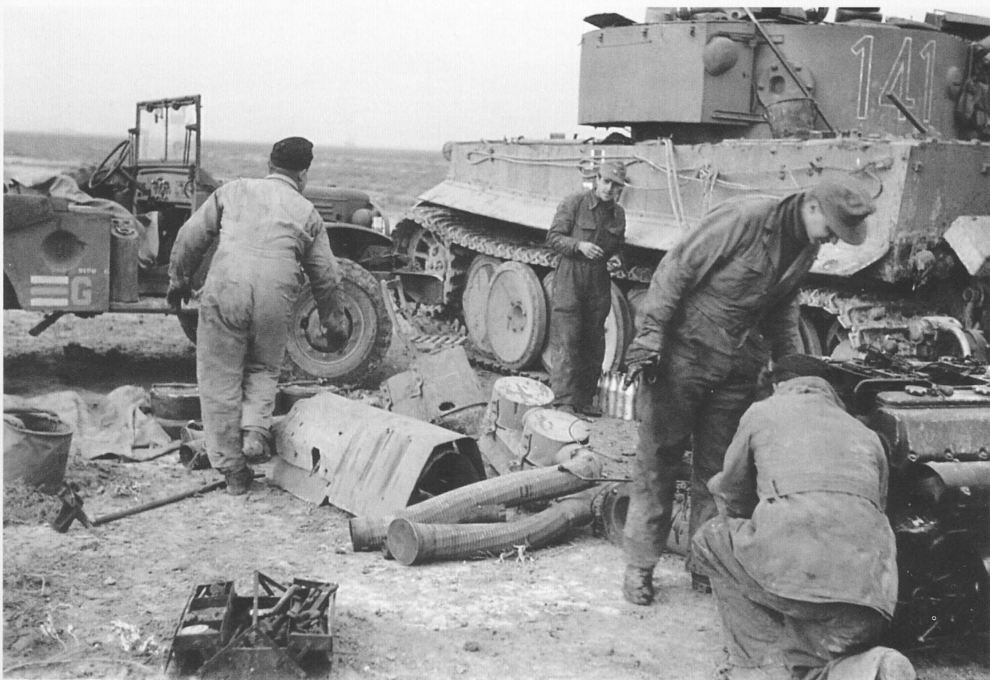
The Feifel pre-filters, seen here disconnected in the centre, were installed beginning in October 1942. These are of the first type with a simplified model appearing in March 1943. The slotted shrouds over the exhaust silencers are also characteristic of the 1 Kompanie. In the background is a Dodge 4x4 – Ton truck, the direct successor of the Dodge - 3/4 Ton depicted on page 4. (NARA)
